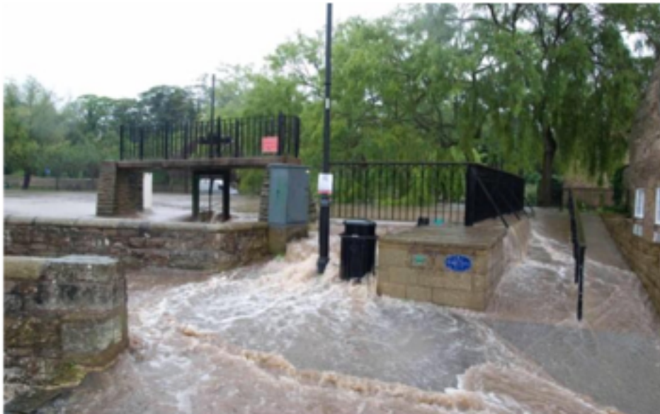
Sluice gate Tickhill Mill Dam, Lindrick, prior to improvements
